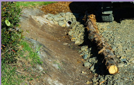
Improvements have been made to the roads, including spoon drains, a culvert and extensions down to pod B.
