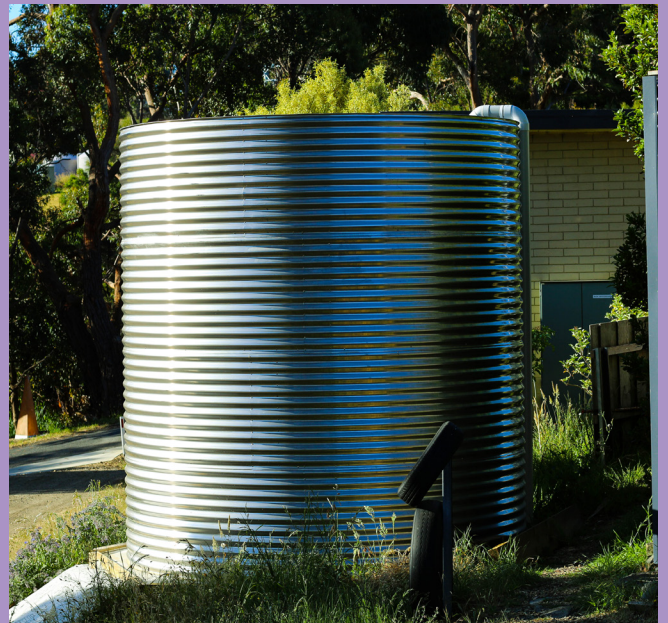
Our water storage capacity was increased when Lot 14 installed a new 23,398 litre stainless steel tank, thank you Sharada and Tony! A new pipe was also installed so that the overflow from the new tank, along with the rainwater from Units 6 and 7 is now directed to Tank 4 which overflowed during the spring rains!
